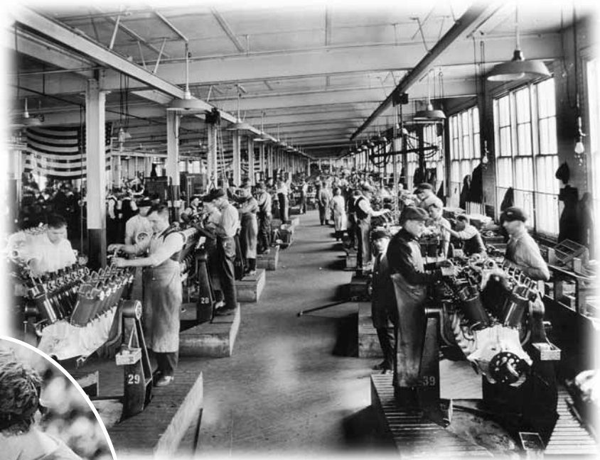
Above: At its peak production in 1918, Lincoln employed about 6000 people producing aircraft engines, including (left) this World War I version of Rosie the Riveter, seen welding Liberty engine water jackets. A great number of women were employed in manufacturing businesses during the war due to the shortage of men. Photo courtesy of NAHC, Detroit Public Library.
