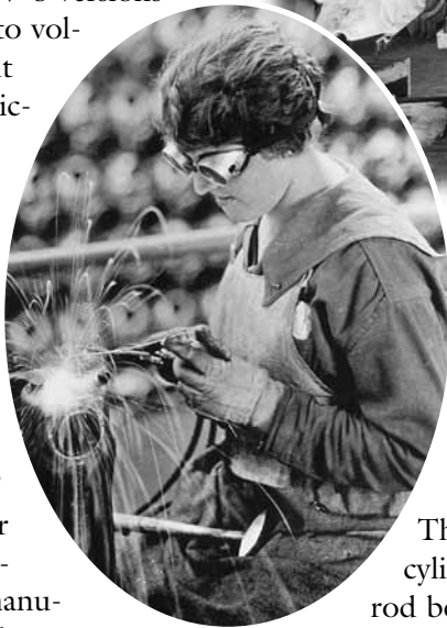
Above: At its peak production in 1918, Lincoln employed about 6000 people producing aircraft engines, including (left) this World War I version of Rosie the Riveter, seen welding Liberty engine water jackets. A great number of women were employed in manufacturing businesses during the war due to the shortage of men. Photo courtesy of NAHC, Detroit Public Library.
