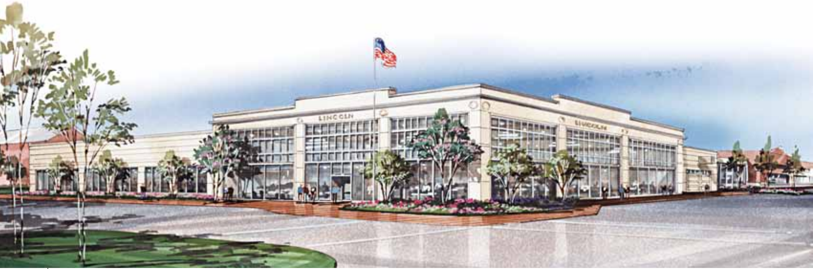
■ When it is completed later this year, the Lincoln Motor Car Heritage Museum, in a building designed by Steven R. Bosch, will take its place among several new marque-oriented museum and research facilities in the architectural image and likeness of historic auto dealership buildings on the campus of the Gilmore Car Museum north of Kalamazoo, Michigan—a mecca for Lincoln lovers from all eras. Architectural rendering by Randy Mytar.
