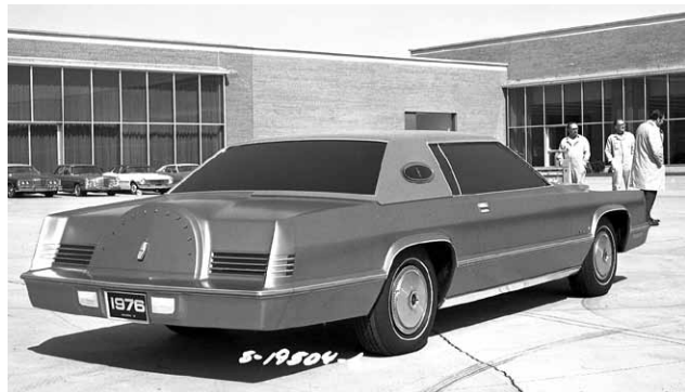
■ Left: This undated photo of a proposed larger Mark V was taken in the courtyard of the Design Center. The taillight proposal on this car was soon changed. Note also, that the proposed production date on the license tag of this Mark V is 1976. Right: Taillights that went over the tops of the fenders first appear in January 1974. They were ultimately removed because Lincoln’s chief engineer thought they could be broken too easily when the trunk was being used.
