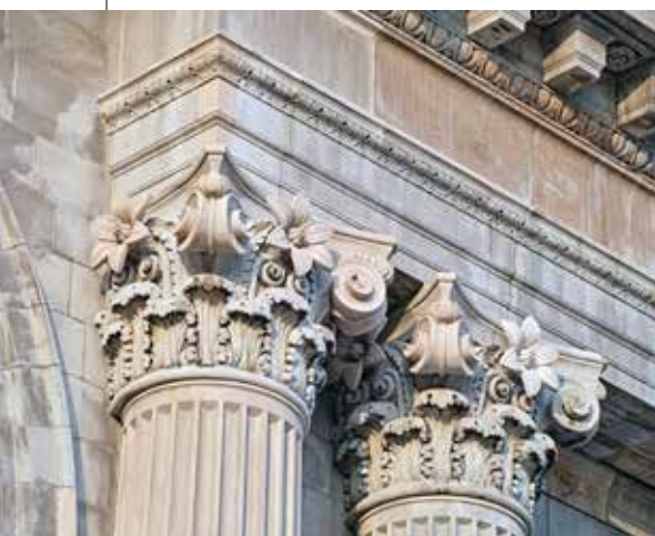
■ The Corinthian columns flanking the building's entrance have been painstakingly rejuvenated, with missing or broken elements re-created from scratch by talented artisans.
